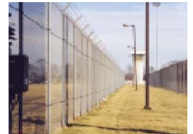
Appropriate perimeter protection
